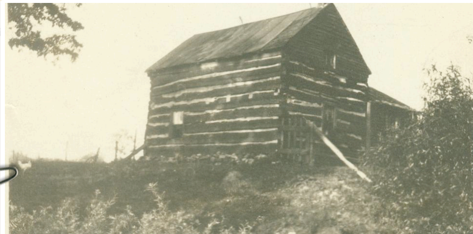
Kuhn Cabin, once located in Newport Township, was associated with the Underground Railroad.
